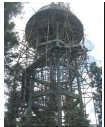
CONSTRUCTION OF OVERHEAD TANK
