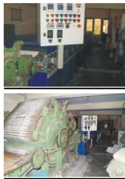
PLASMA PLANT INSTALLED AT HIFEED CAMPUS
