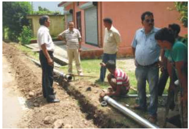
BORING WORK UNDER SWAJAL PROJECT
