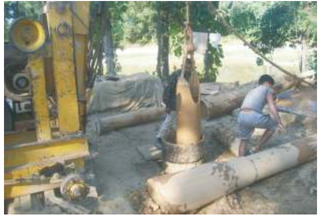
BORING WORK UNDER SWAJAL PROJECT
