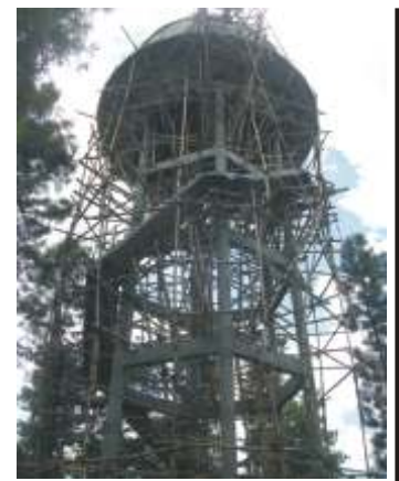
CONSTRUCTION OF OVERHEAD TANK
