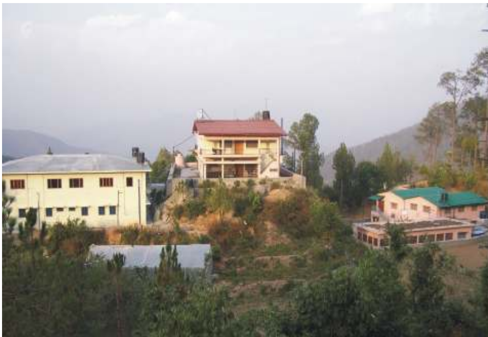
HIFEED CAMPUS AT RANICHAURI
