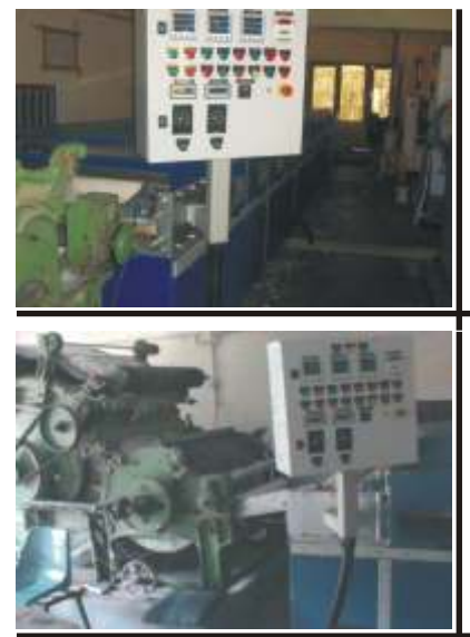
PLASMA PLANT INSTALLED AT HIFEED CAMPUS
