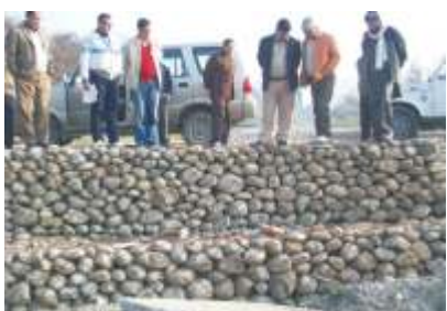
MGNREGA SITE VERIFICATION IN SAMBA DISTRICT IN J&K
