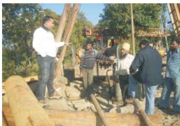
BORING OF TUBEWELL UNDER SWAJAL PROJECT
