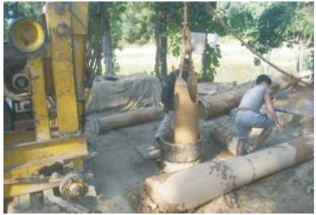
BORING WORK UNDER SWAJAL PROJECT
