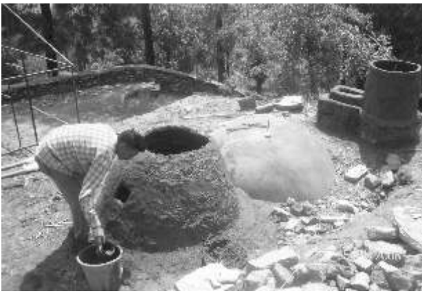
CONSTRUCTION OF RAINWATER HARVESTING TANK
