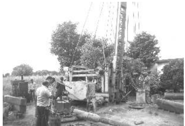
BORING OF TUBEWELL UNDER THE PROJECT
