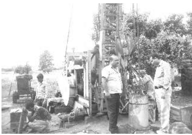
BORING WORK UNDER THE PROJECT
