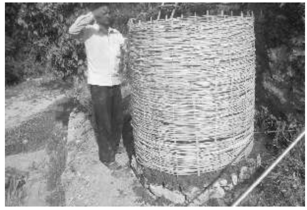
CONSTRUCTION OF SHRAMI K BANDHU BIOGAS PLANT
