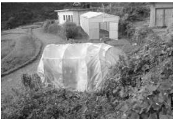
CONSTRUCTION OF LOW COST POLY TUNNEL
