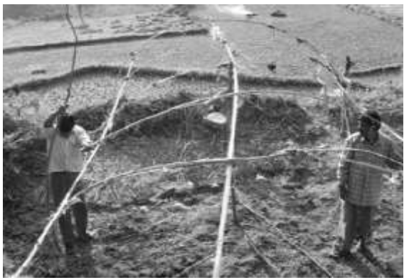
CONSTRUCTION OF LOW COST POLY TUNNEL
