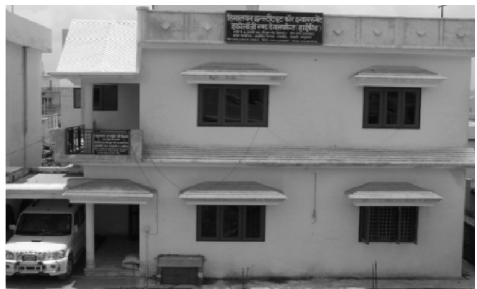
ADMINISTRATIVE OFFICE AT DEHRADUN
