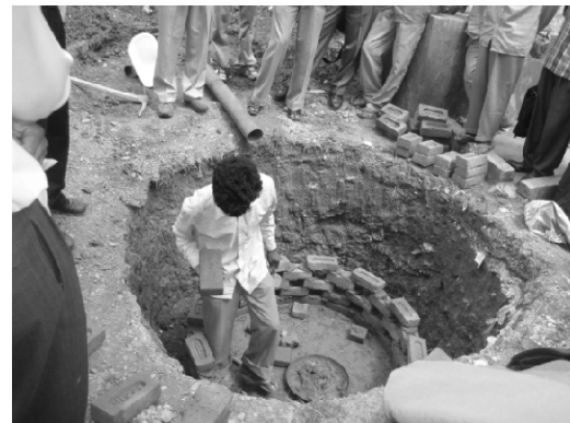
CONSTRUCTION OF LOW COST SANITARY LATRINE
