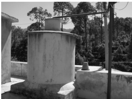
ROOF TOP RAIN WATER HARVESTING TANKS
