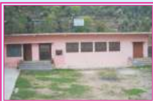
PRODUCTION CENTRE OF HIFEED AT RANICHAURI
