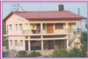
TECHNOLOGY RESOURCE CENTRE OF HIFEED AT RANICHAURI
