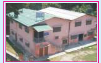
COMMON FACILITY CENTRE OF HIFEED AT RANICHAURI
