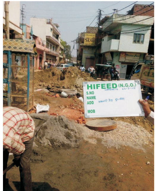
Verification of Sewer Connection, Namami Gange Program, (U.P.)
