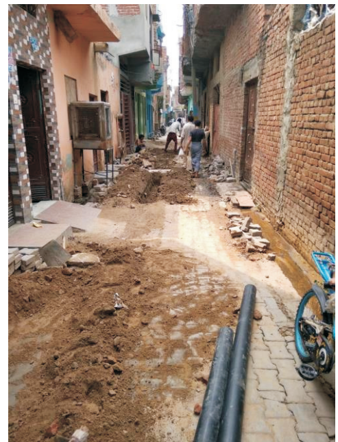
Lying of Sewer Lines, Muzaffarnagar (U.P.)
