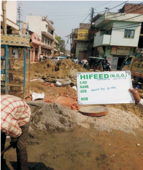
Verification of Sewer Connections, Namami Gange Program at Ghaziabad, U.P.
