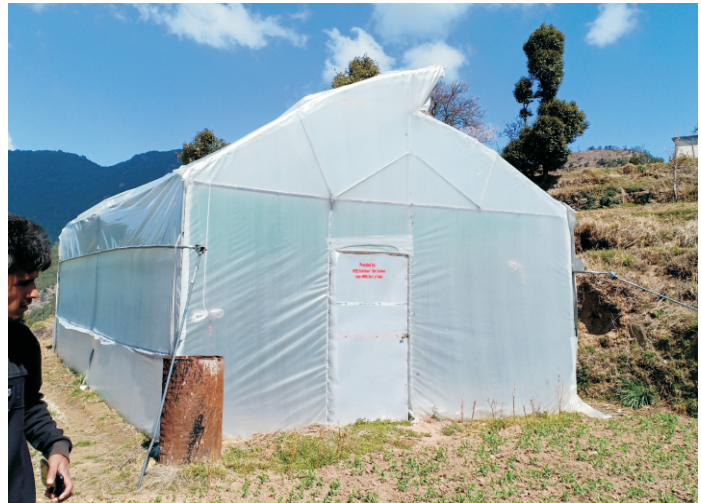
Naturally Ventilated Poly House
