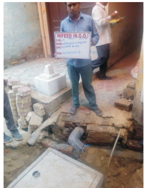
Verification of Sewer Connections, Namami Gange Program at Muzaffar Nagar, U.P.
