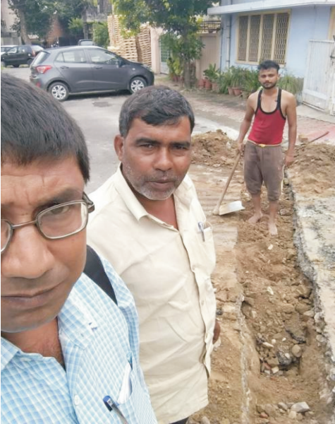
Verification of Sewer Connections, Namami Gange Program at Meerut, U.P.
