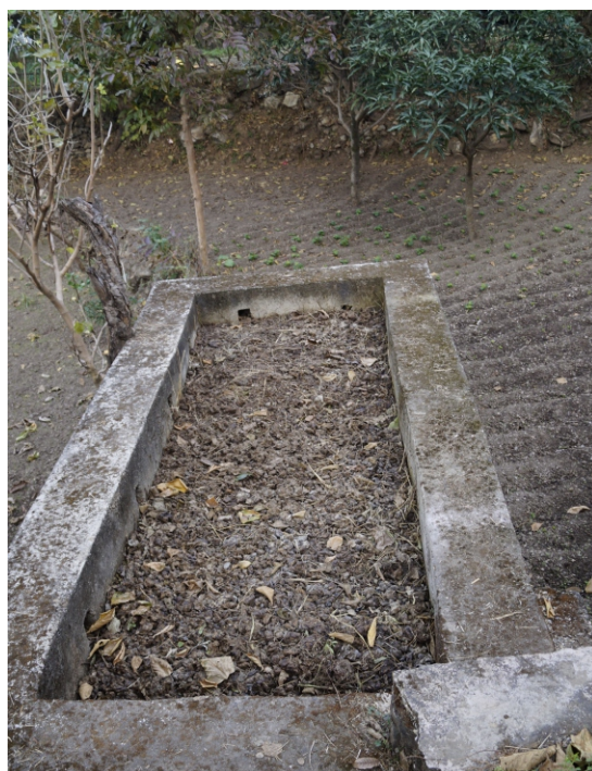
VERMI COMPOST PIT CONSTRUCTED AT FARMER'S FIELD
