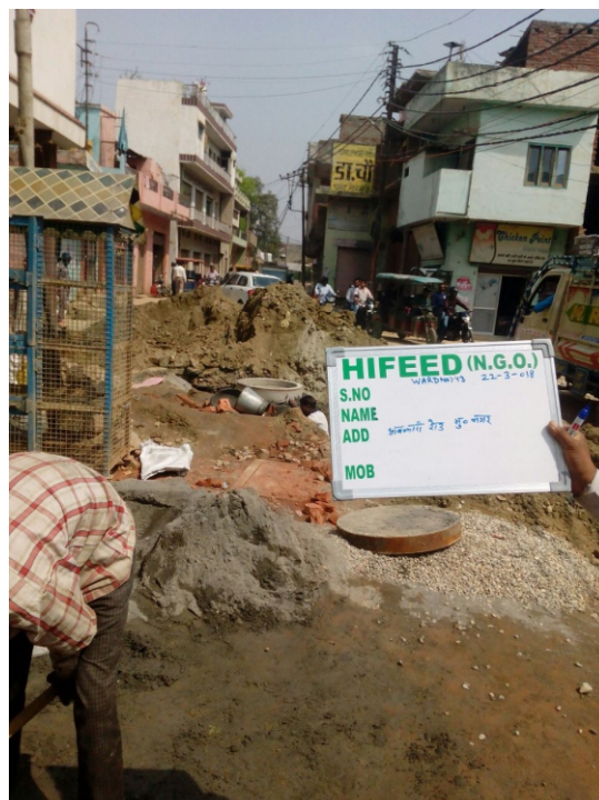
CONSTRUCTION OF SEWER LINES IN MUZAFFAR NAGAR CITY, U.P.
