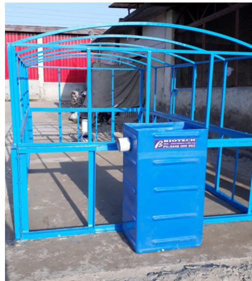
FRAMED STRUCTURE OF BIODIGESTER
