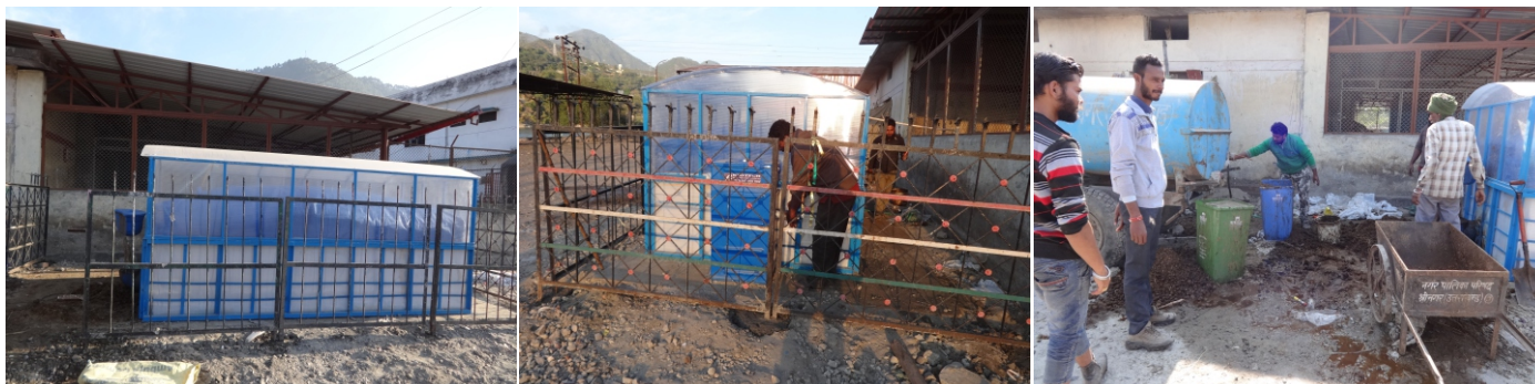
INSTALLATION OF HIGH RATE MODULAR BIODIGESTER AT SRINAGAR
