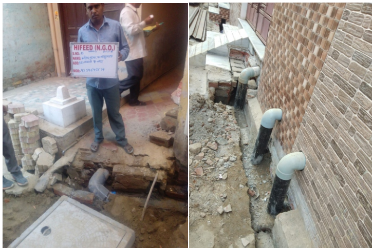
CONSTRUCTION OF SEWER LINES IN MUZAFFAR NAGAR CITY, U.P.
