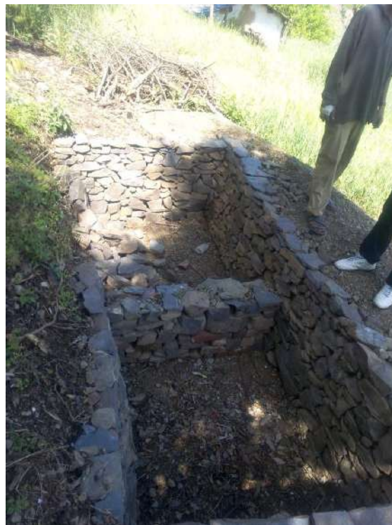
VERMI COMPOST PIT CONSTRUCTED AT FARMER'S FIELD
