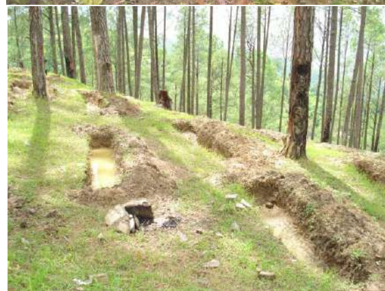
WATER HARVESTING TANK CONSTRUCTED UNDER THE PROJECT
