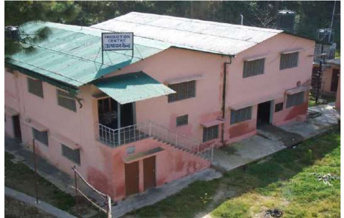
COMMON FACILITY CENTER OF HIFEED AT RANICHAURI
