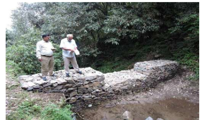
CHECK DAM CONSTRUCTED UNDER THE PROJECT
