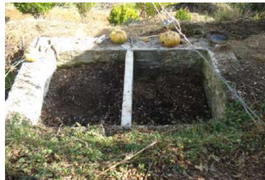
VERMI COMPOST PIT CONSTRUCTED UNDER THE PROJECT
